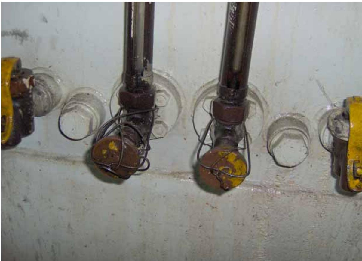
Similar to the spring loaded oil tank sight glass valves, it is also seemingly forgotten why double bottom tank sounding pipes are fitted with self closing weighted cocks, and these are also found gagged open or disconnected.
